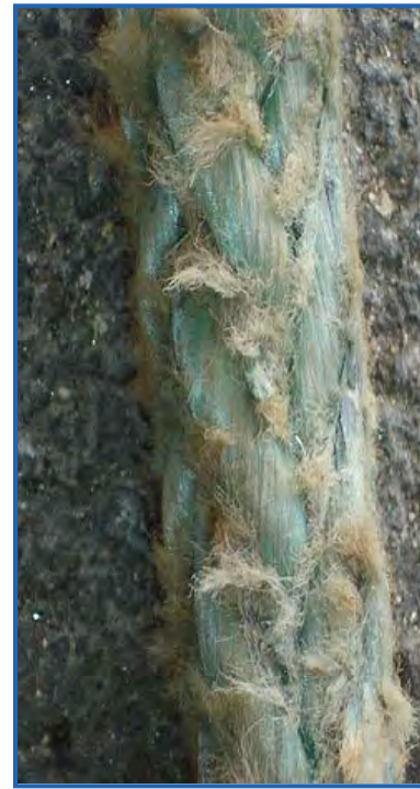
Figure 10d Rope with Wear and Burned Fibers
