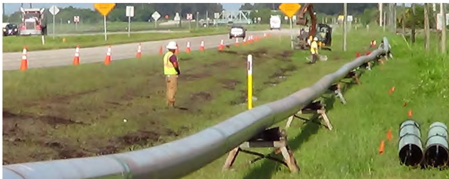
Typical Drill string welded and coated, prepped for pullback
