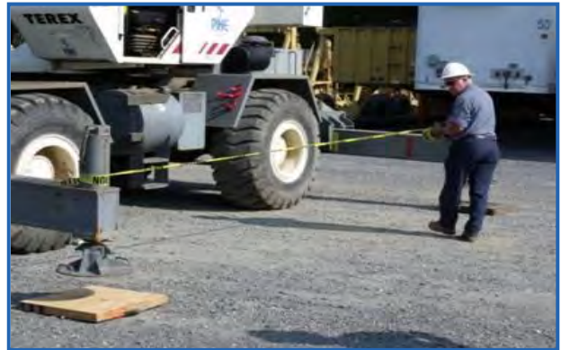
Figure 10h Barricading Swing Path
