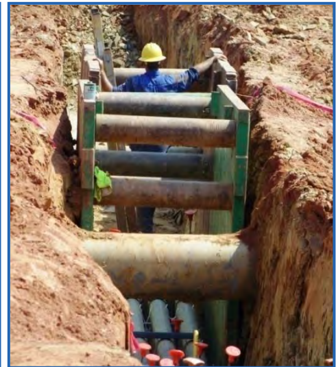
Figure 6d Shoring Protective System
