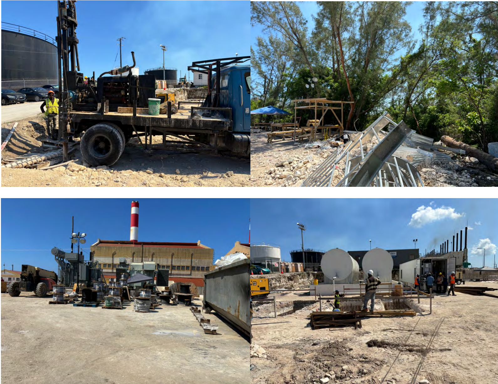
Figure 2-8: Current LNG-to-Power Project, Phase 1 site
