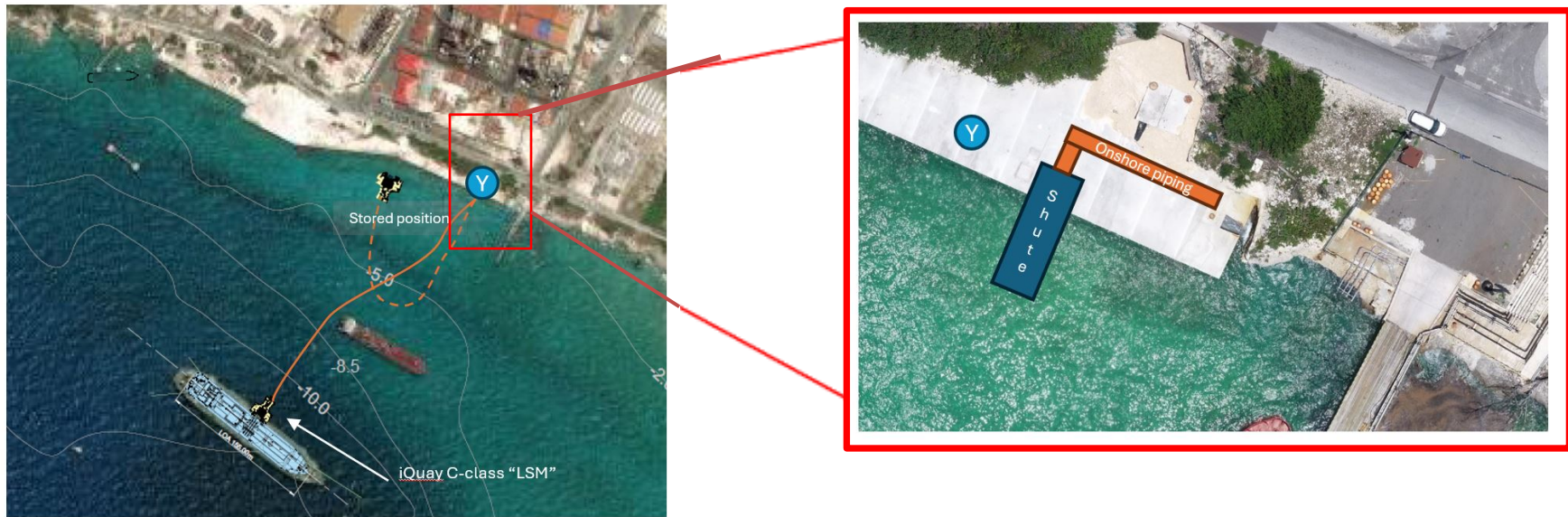
Figure 2-2: Floating econnect system
